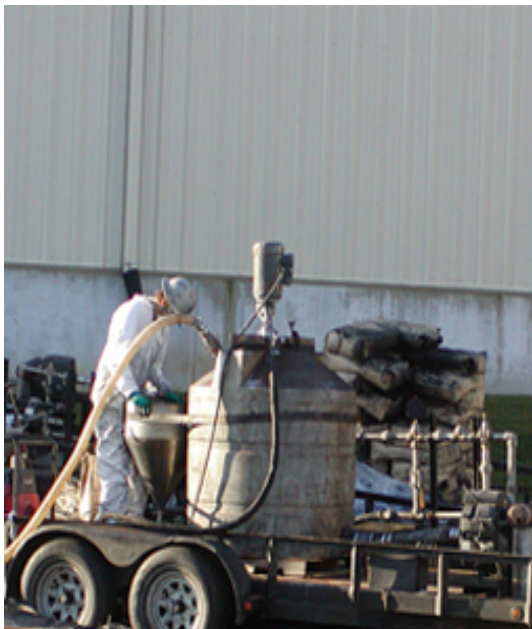
Site photo during injections
