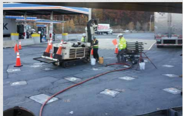
FIGURE 2. PROJECT PHOTOGRAPH SHOWING INJECTION LOCATIONS
